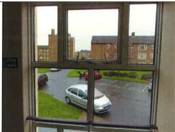
Opening window in stairwell
